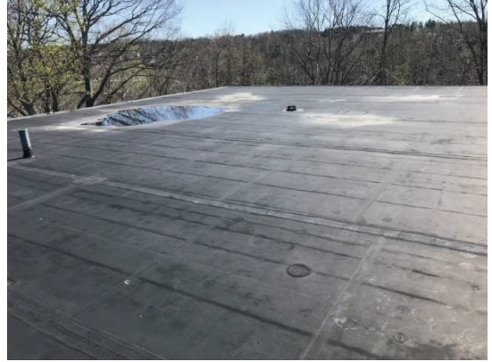
Exterior view - roof
