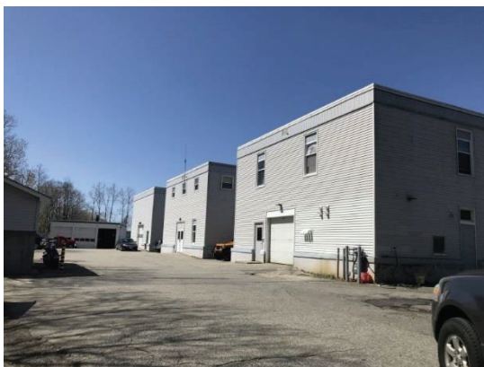
Exterior view - rear/eastern elevation
