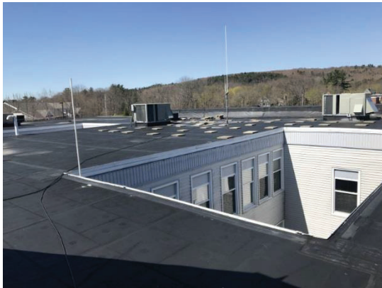
Exterior view - roof
