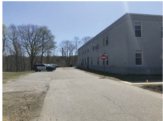
Exterior view - side/northern elevation
