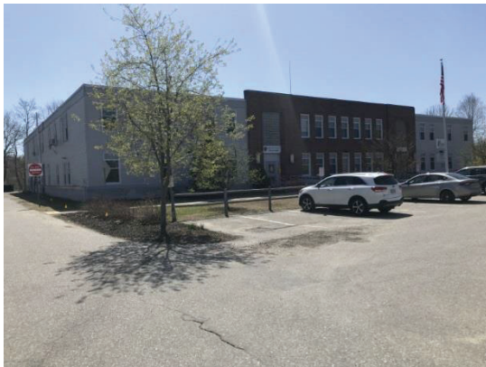
Exterior view - front/western elevation
