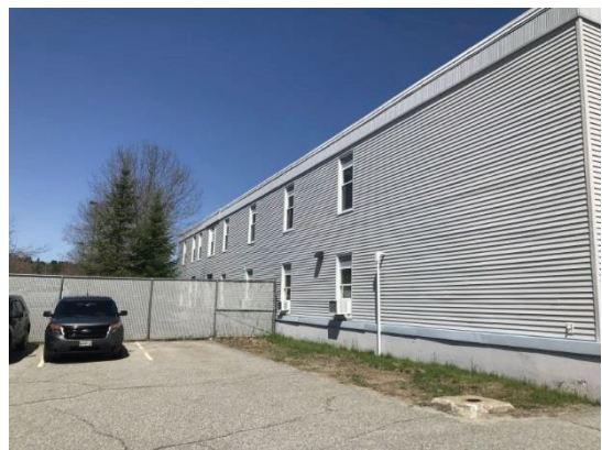
Exterior view - side/southern elevation
