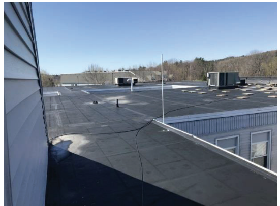
Exterior view - roof
