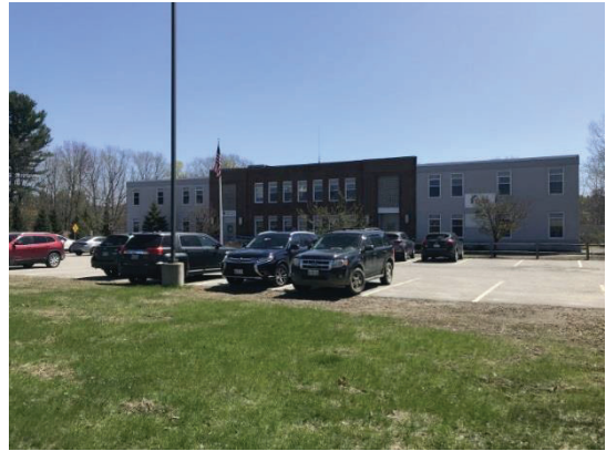
Exterior view - front/western elevation
