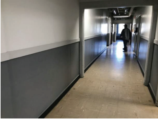
Interior view - typical corridor
